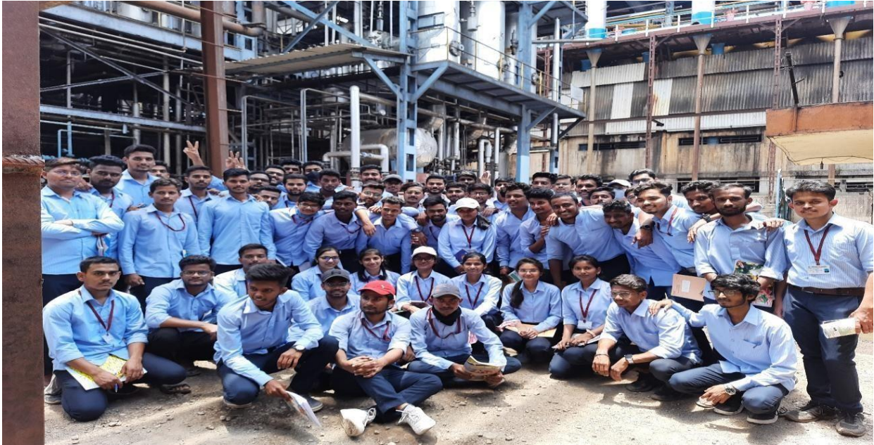
Distillery plant at Rajarambapu Sugar Industry, Sakharale, Islampur., Tal. Walwa, Dist. Sangli.
