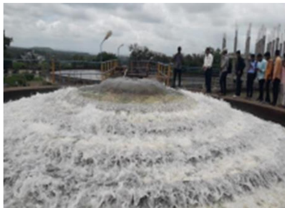
Photo No.1 Aeration Fountain
